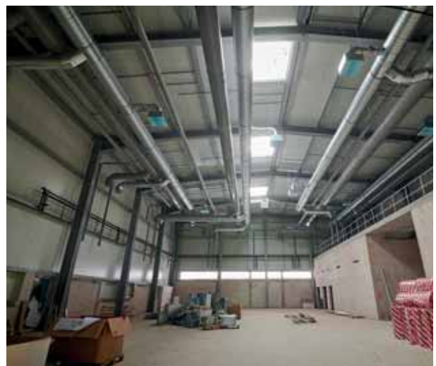
The Transfer Technical Center under construction.
